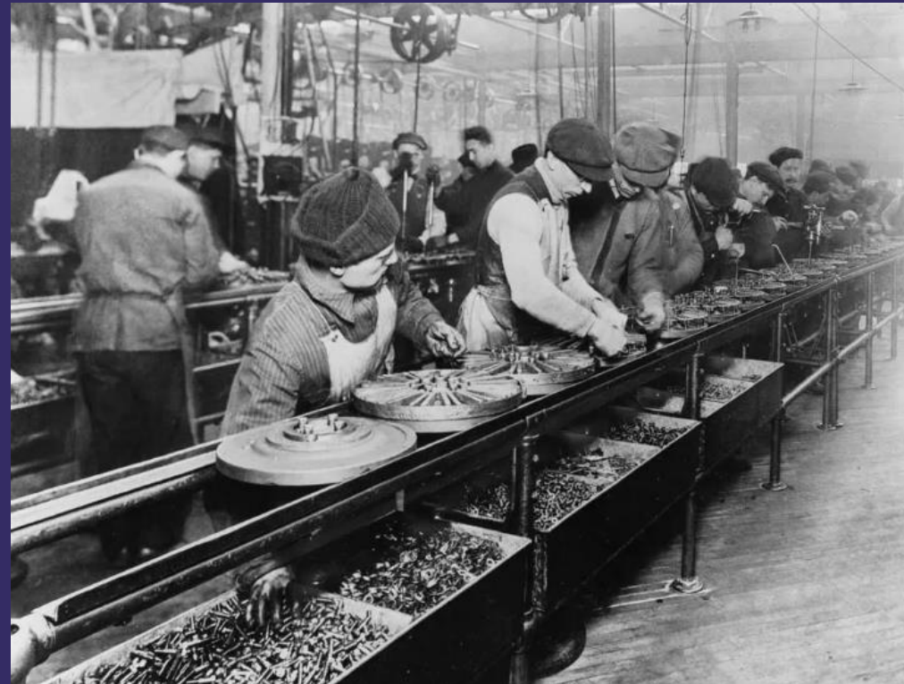
Electric assembly line
